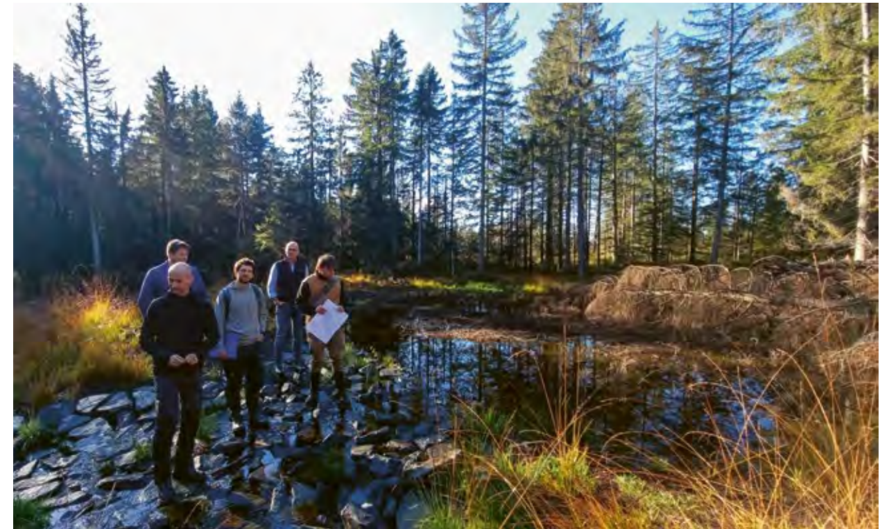
Final inspection of an overflow protection drainage
